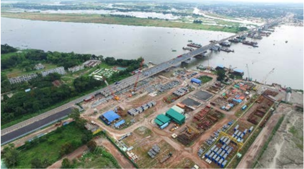
Gumti Bridge construction status (June 2018)
